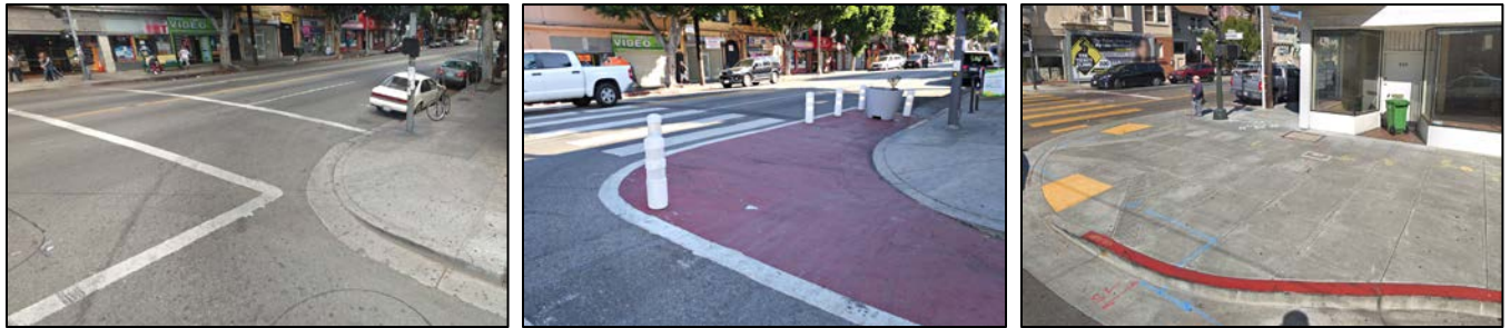
Figure 1. Intersection of St. Louis and César Chávez Avenue before (far left) and after (middle) installation of a painted curb extension, compared to a concrete curb extension (far right).
